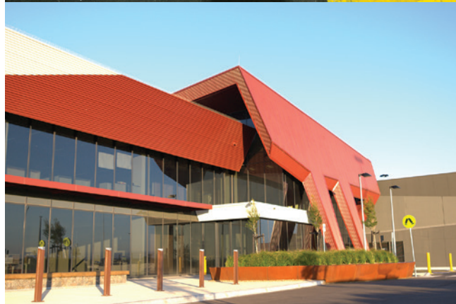
MMA administration building and conference centre at the new Market at Epping.
