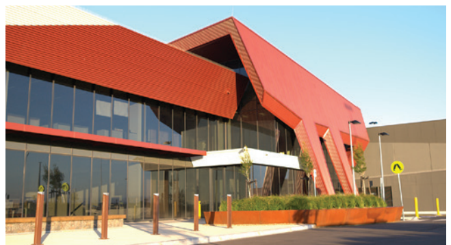
MMA Administration building and Conference Centre at the new market at Epping.
